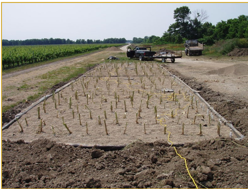
10 - Constructed wetland, construction (above) and after 2 years (below).
